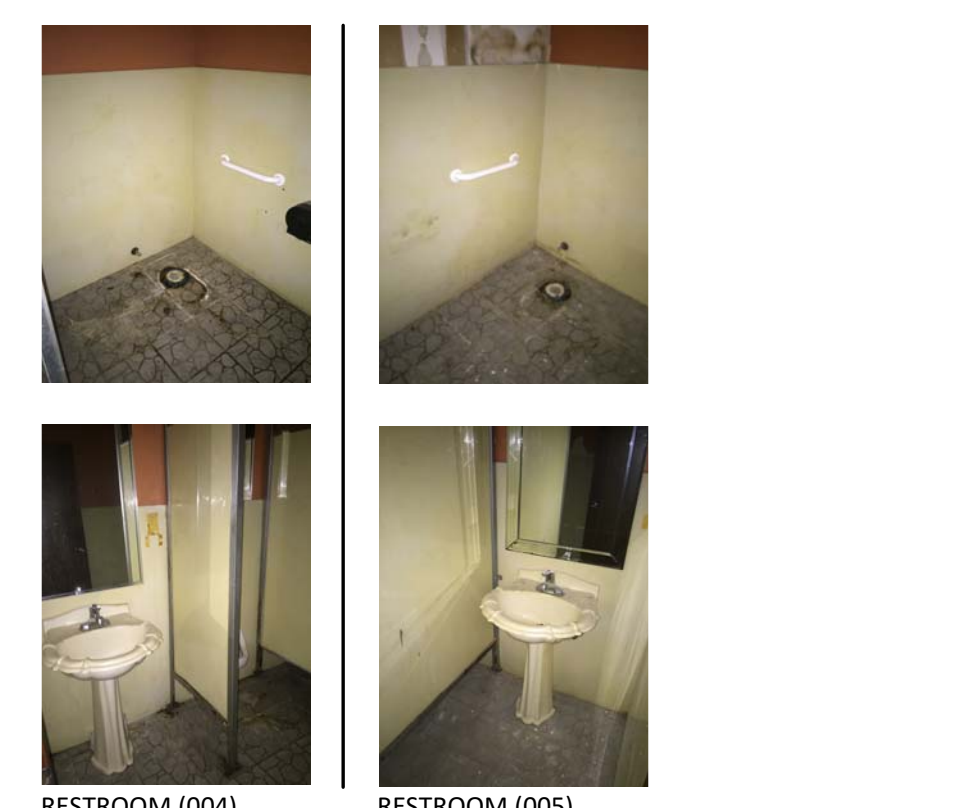
RESTROOM (004) RESTROOM (005) 1 RESTROOM COMPLIANCE (PHOTOS) NOT TO SCALE
